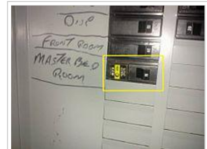
This AFCI (the circuit breaker with the yellow label) is an older generation AFCI circuit breaker. The current (as of 2013) devices are referred to as "combination type" and usually appear with a green label.
